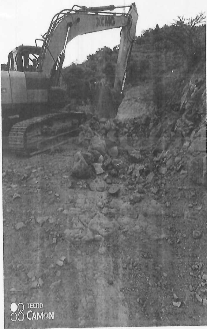
H3 Ogongo Kipasi Road in Lambwe Ward
