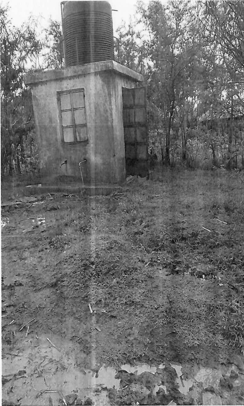
Water bore hole in Ndihiwa with broken taps due to lack of community maintenance
